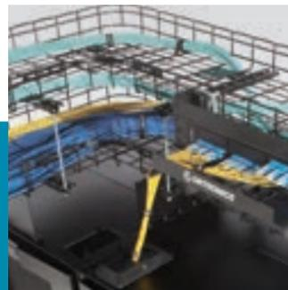
Multiple cable pathways are compact with easy access to cables.
